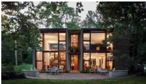
Louis I. Kahn, Margaret Esherick House , Rear Facade, 1959 – 1962; restored 2014 – 2016, k YODER design. Photo: © Jeffrey Totaro Photography.
