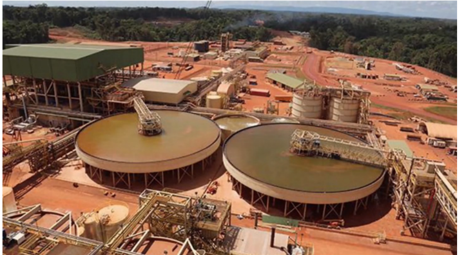
Merian Goldmine of Surgold, Newmont Suriname. Photo courtesy of ATV-Networks.
